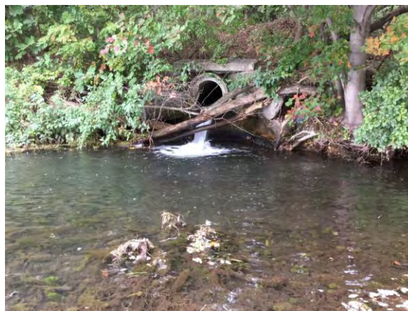
Outfall near Crosstown Trail.
