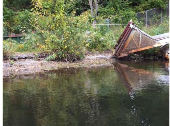
Weed removal equipment storage area.
