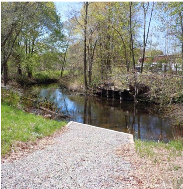
Stabilized kayak/canoe launch using wood and stone.
