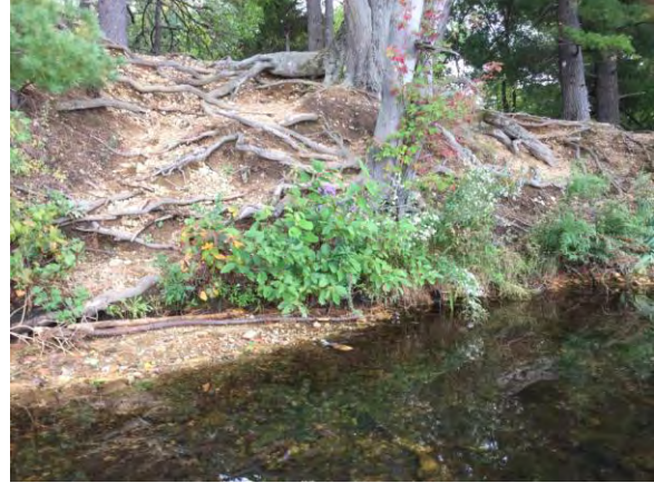
Steep and eroded pond access location.
