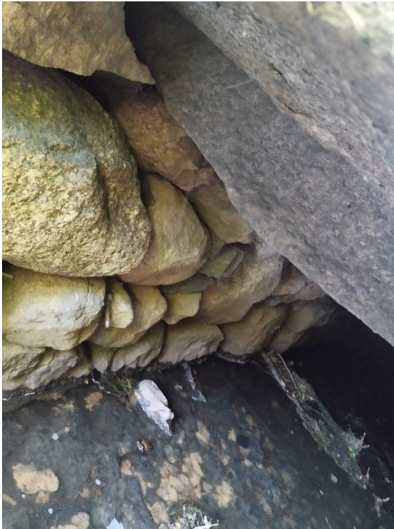
Photos No. 9 and 10 – View of boulders placed along box culvert walls
