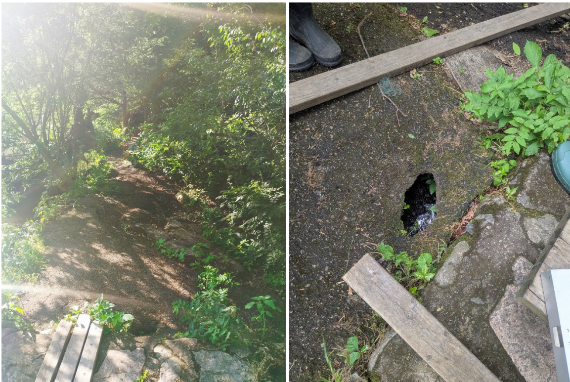
Photos No. 1 and 2 – Area north of the culvert where temporary fix and erosion were observed.
