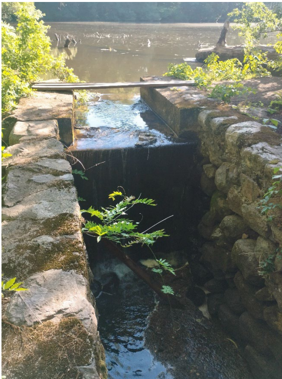
Photos No. 7 and 8 – View of the broad crested weir and spillway, as well as box culvert stone cover.
