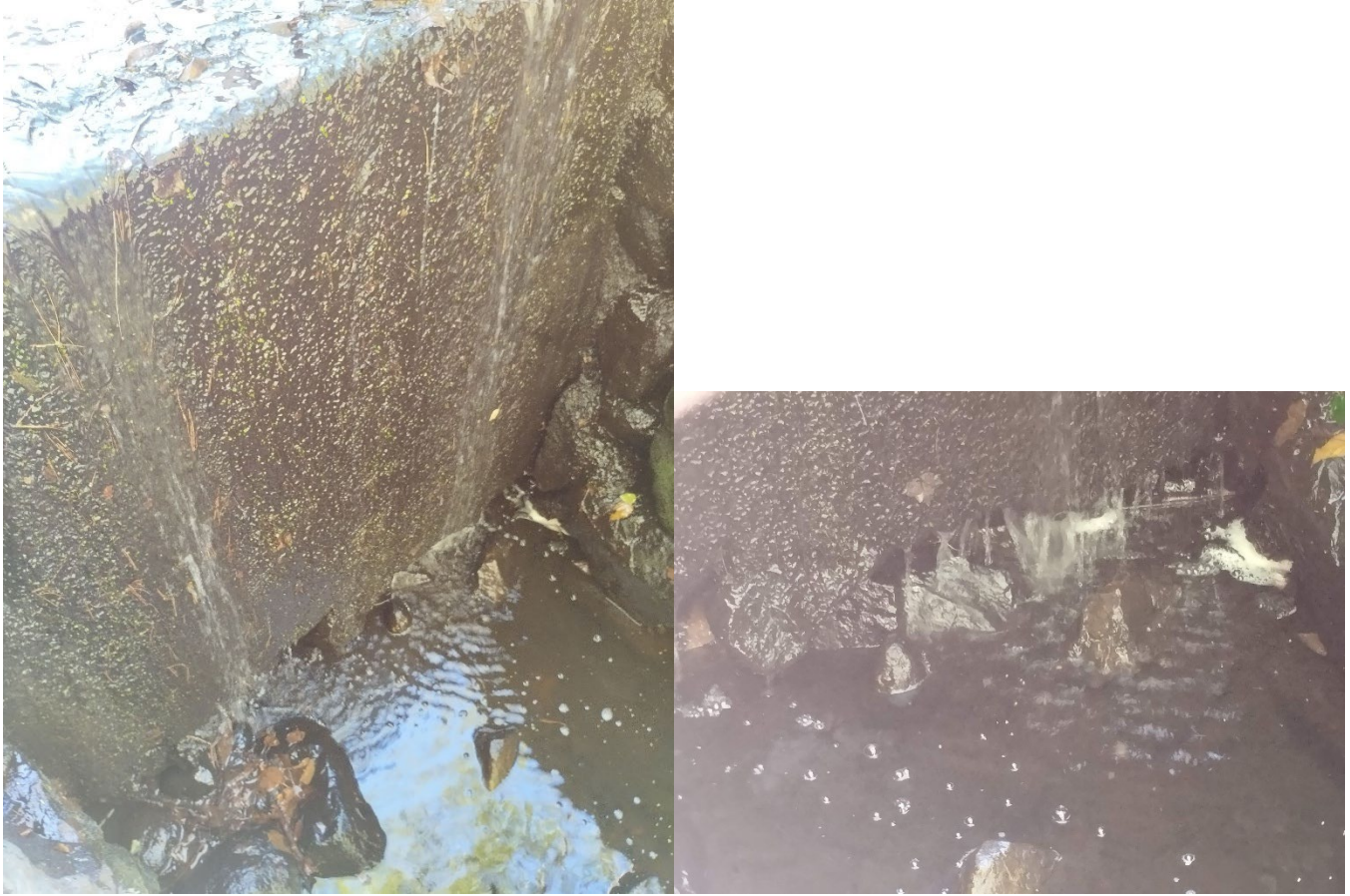
Photos No. 13 and 14 – Views of the base of the spillway showing erosion of material from the base of the structure.
