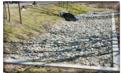
Image: Infiltration trench with piped inflow. Source: MA Stormwater Handbook.
