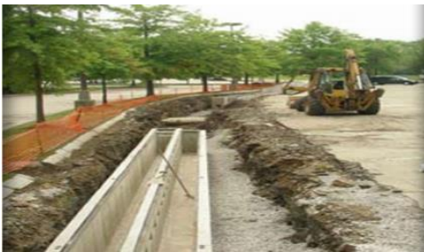
Image: Construction of a sand filter. Source: MA Stormwater Handbook
