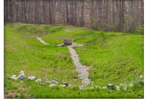
Image: Dry detention basin with impervious channels. Source: MA Stormwater Handbook
