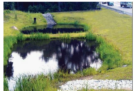
Image: Wet Pond and Forebay. Source: Mass Highway Storm Water Handbook
