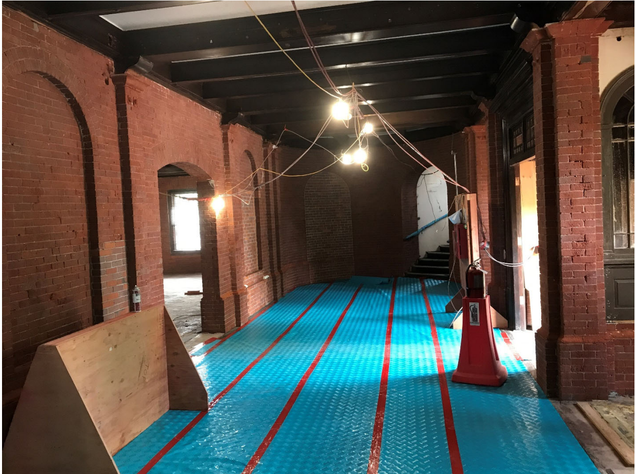
Town Hall's front entry with the paint removed from the bricks. Photo courtesy of Town of Wellesley
