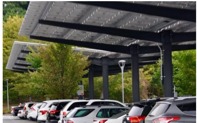
Image of canopy supported PV array
