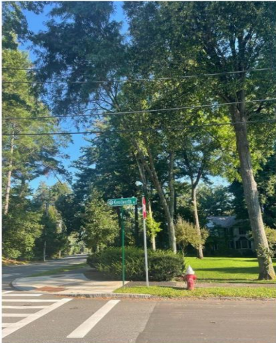
Asphalt to granite curb & ADA ramp
