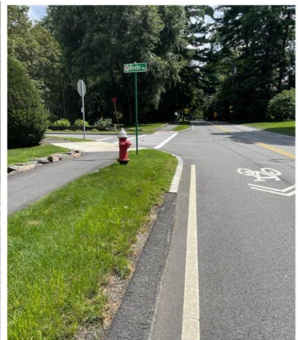
Asphalt to granite curb with hydrant & bicycle sharrow
