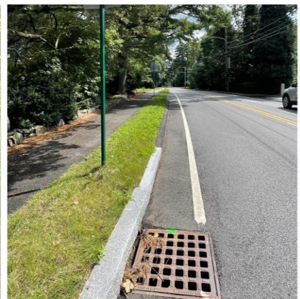
Asphalt to granite curb at catch basin
