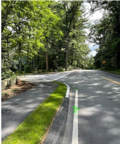
Asphalt to granite curb at corner
