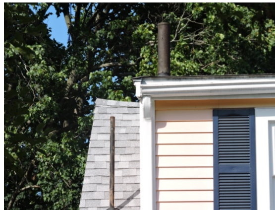
Plumbing vents must be located above bathrooms but should be colored to be minimally visible.
