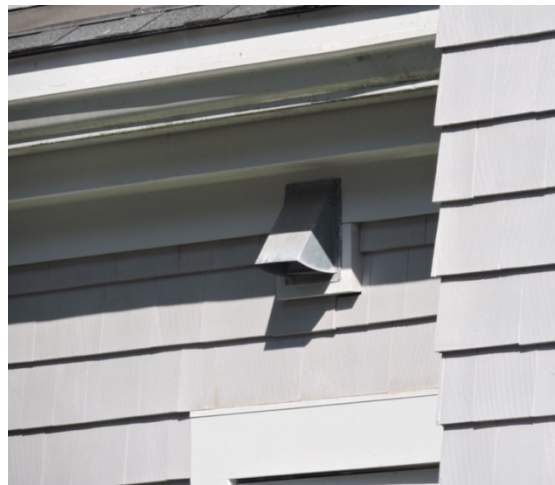
Mechanical installations such as electrical boxes and dryer vents should be located on side and rear facades and should be minimally visible from the street.
