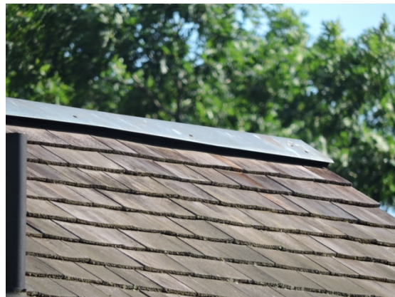
At least one wood shingle roof remains in the historic district. It has a metal ridge cap/vent, not historically accurate but acceptable for function and longevity.
