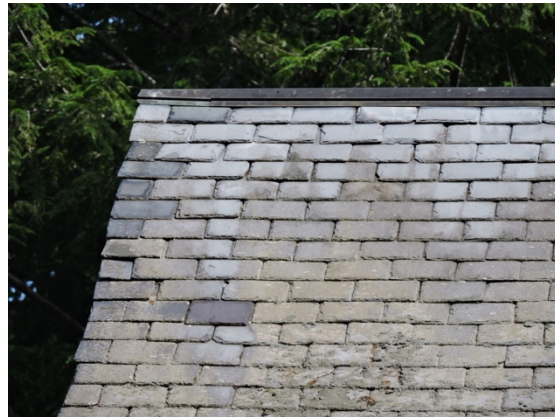
This slate roof has a copper ridge cap. Copper in the water washing down from the cap has killed lichen that is seen growing on the slates in the lower portion of the image. The dark grey slates are replacement pieces – a better color match might have been possible.
