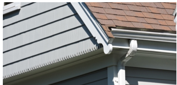
Contemporary K-style (molding shaped) gutters have been installed inside of decorative barge boards at the gable ends.
