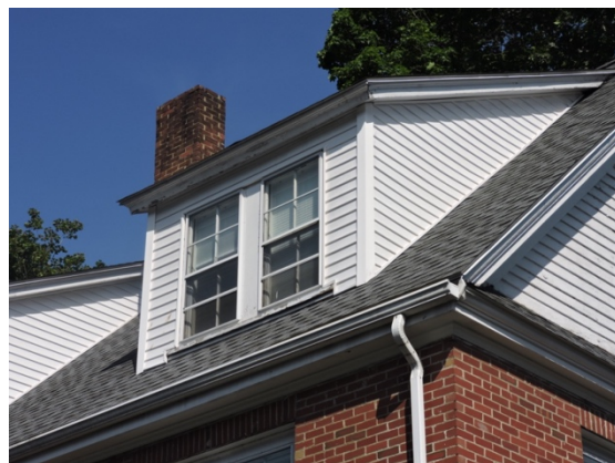
These dormers appear to have been added to the building to make the attic level habitable.
