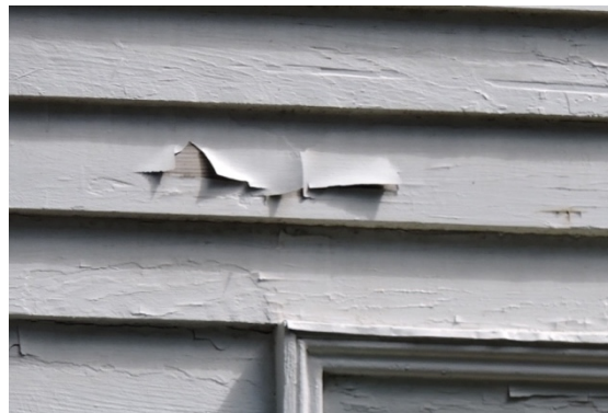
Painted coatings are necessary to protect wood. Peeling paint is often caused by water vapor moving from the interior to the exterior of the building.
