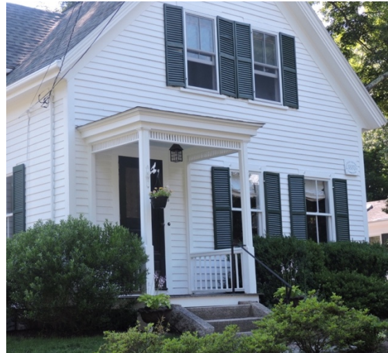
Entrance porch with a flat roof, simple wood structure, railings, wood deck, and stone steps.
