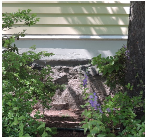
Wood detailing can be susceptible to water penetration and deterioration, such as at this drip edge and trim at the base of a clapboard wall.
