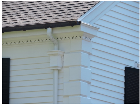
Fine detailing of a roof edge – half-round copper gutter, downspout matching the color of the wood eave and walls, and scupper box.
