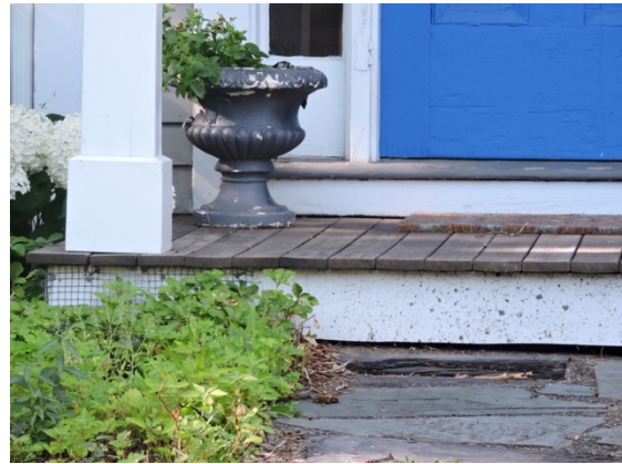
Wood porch flooring and related elements are exposed to the weather and susceptible to deterioration.
