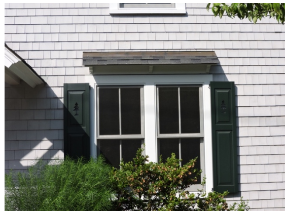
These shutters do not match the size of the historic window opening and could not be operable.
