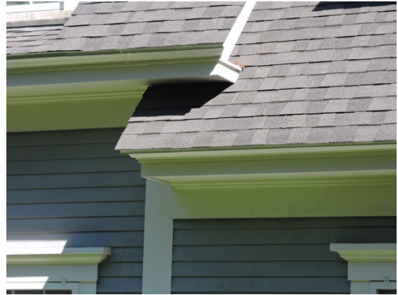
Asphalt shingles are in use throughout the historic district and are easily adaptable to complex roof intersections such as these. This roof has no gutters, a common historic condition.
