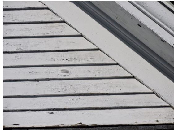
This siding shows some indication of peeling. A small metal vent has been installed to allow interior moisture to escape, rather than allowing it to move through the wood causing the paint to fail.
