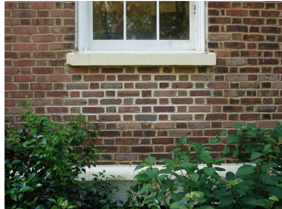
The repointing below the window in this historic wall does not match the color, texture, or tooling of the historic mortar to the right and left.
