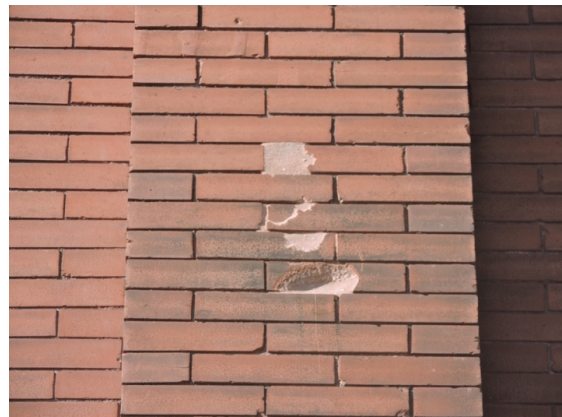
The surfaces of these bricks have spalled.
