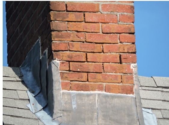
Chimneys are the most frequently present brick features in wood buildings within the Cottage Street Historic District. Difficult to access, this brick chimney has open joints which will absorb water.
