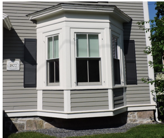
Stone foundation of a wood framed vernacular building within the Cottage Street Historic District.
