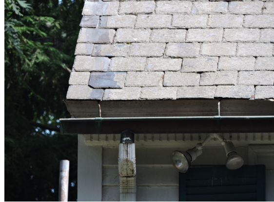
Copper is a common historic material used for roofing, gutters, and downspouts and should be retained whenever possible.
