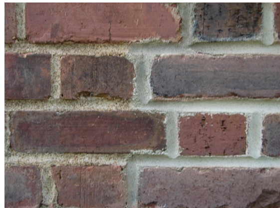
Detail of repointed joints showing modern grey mortar to the right that does not match the rich brown color and texture of the historic sand mortar to the left.
