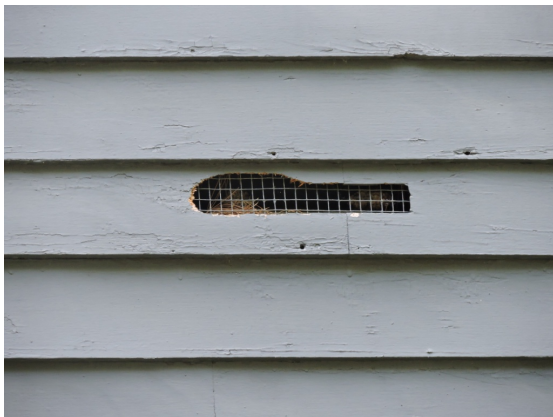
This hole in historic wood siding may have been intentionally cut as a vent, but it has been widened by chewing animals and nesting material can be seen inside.
