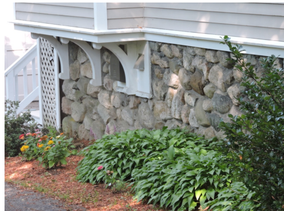
A rubble stone foundation wall at a house within the district.
