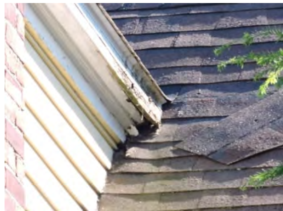
The fascia and soffit boards of this cornice have rot due to moisture drawn from contact with the roofing. The hole in the soffit on the underside of the cornice is probably an entranceway for squirrels.
