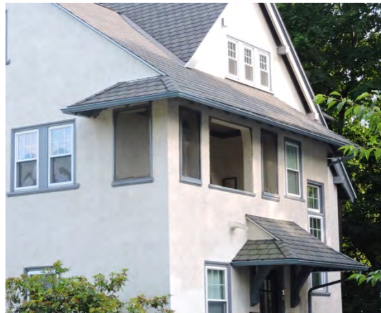
Stucco is present but in limited use within the historic district, but contemporary asphalt shingles are widely used, reasonably priced, and easily adaptable to a wide variety of forms and conditions.
