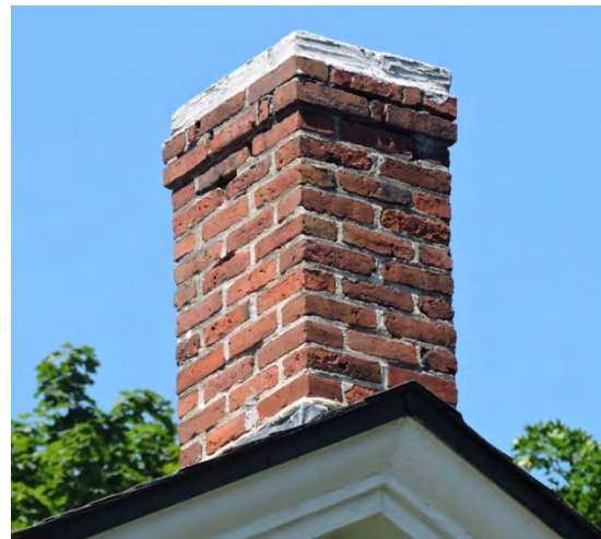
The bricks in this chimney show their age – some are chipped and slightly spalled. They need not be repaired or replaced, however, if they do not threaten the masonry as a whole.
