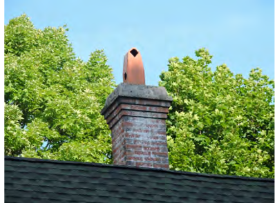
This chimney within the historic district appears to have a custom stone cap with a terra cotta flue cap.
