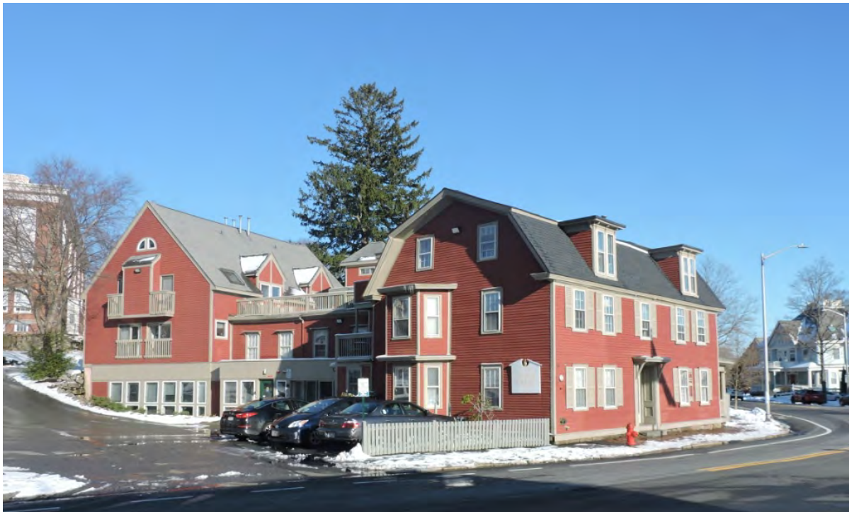
This 18 th century historic residence in Beverly, MA was converted to commercial office use with a large but compatible addition to the rear. Though large, the addition modulates reasonably in form in relation to the historic residence. It uses matching materials and colors but has creative contemporary elements.
