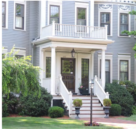
Highly detailed front porch with wood columns, roof balustrade, floor, and steps.
