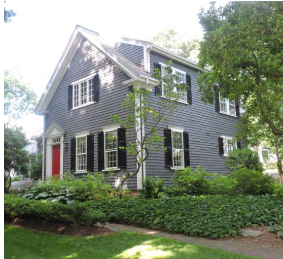
The flush dormer above may be a later addition to make the second floor of the building more usable and has gained historical significance due to its age. New dormers should be set back from the first floor wall plane so that the overall cottage form of the building is better retained.
