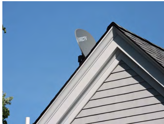
An internet/television dish was installed on the back side of this building's ridgeline so that it is minimally visible from the street.
