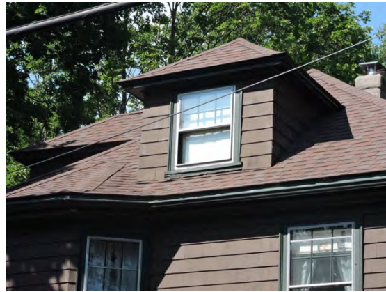
Historic dormer characteristic of the building's period and architectural style.
