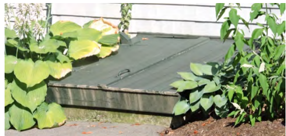
Wood basement areaway door.
