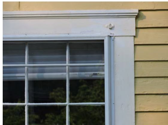
This exterior metal storm window is discretely mounted on the historic window frame, matching its size, and is barely visible.
