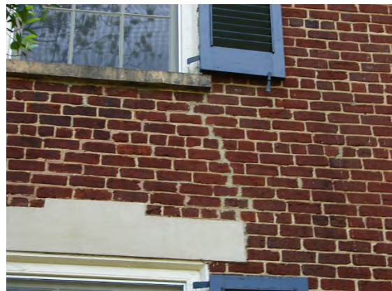
Repair of a structural crack caused by building settlement between the head of the window below and the sill of the window above.
