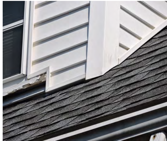
The use of synthetic materials and even aluminum siding, shown here, may be permitted at particularly vulnerable and hard to maintain locations.
