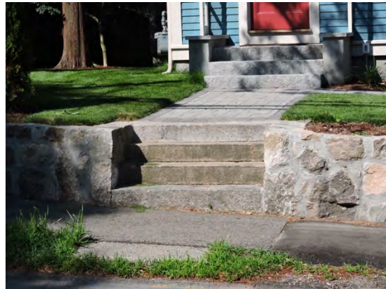
Stone retaining wall and entrance steps.
