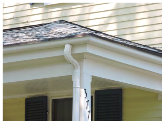
The roofs on this home have built-in wood gutters that are lined with metal, important historic features that have been preserved and maintained.
