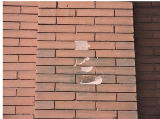
The surfaces of these bricks have spalled.
