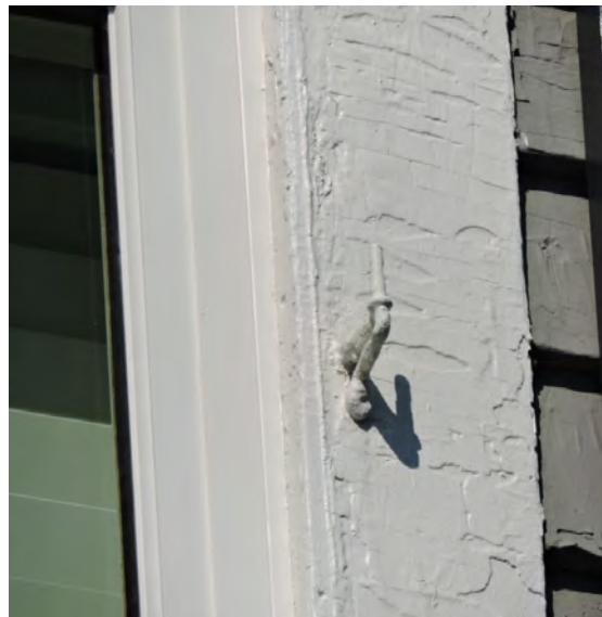
As also discussed in Chapter 7, remnant historic metal features such as this pintle form a late nineteenth century shutter hinge should be preserved whenever possible.
