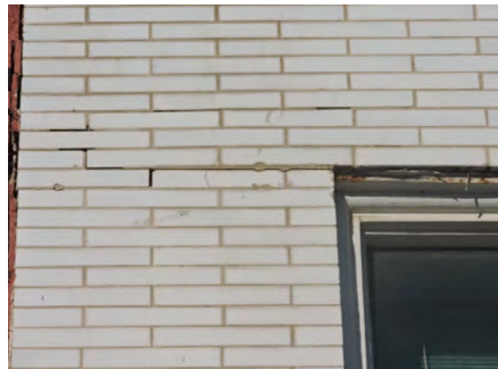
Jacking of a steel lintel at the window to the right has caused cracking of the brick masonry at left.
