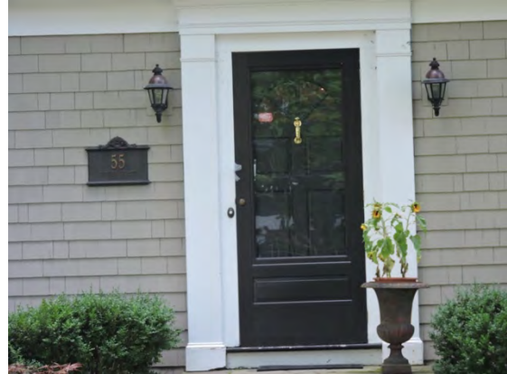
Wood storm door with a large glass panel allowing the historic door behind to be visible. Both are the same color. The glass panel may be replaceable with a screen panel in summer.
