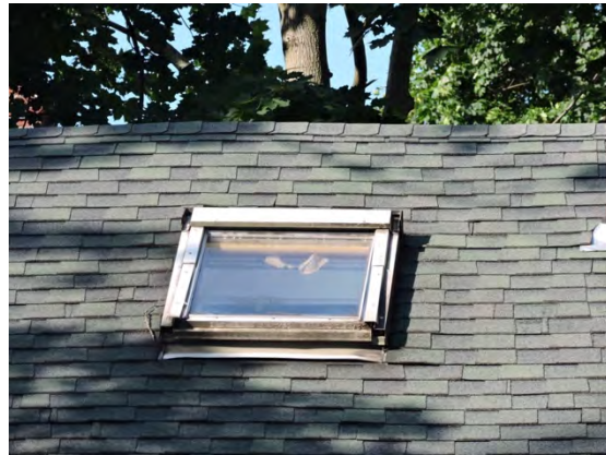
This flat skylight is an appropriate type, but was installed on a primary façade. Its color could have been darker, blending better with the color of adjacent shingles.
