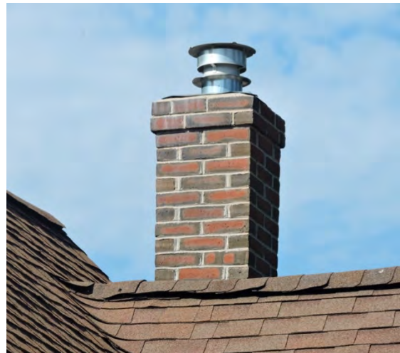
A variety of different types of metal caps have been installed on chimneys within the district, not historic but acceptable for fire safety. This chimney has been rebuilt with brick reasonably similar to the appearance of historic brick.
