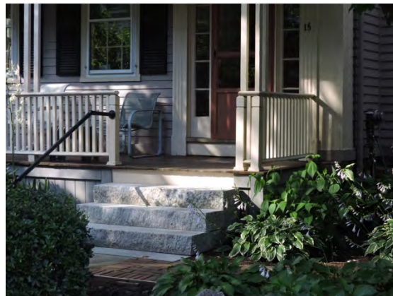
Modern granite steps with smooth treads and rough faced risers have been added to this porch. A black metal handrail has been installed for safety but is minimally visible.
