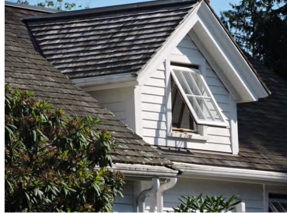
Operable awning window with the screen mounted on the inside.
