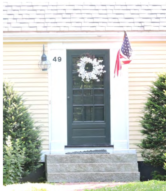
Flush wood doorway with wood side pilasters and crisp stone steps. The storm door has a large glass panel with true divided lights, a preferred treatment. The glass panel may be replaceable with screen panel in summer.
