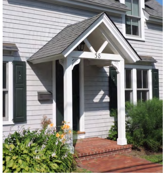
Simple entrance porch with a gable roof structure, decorative structural details, and brick step and deck.
