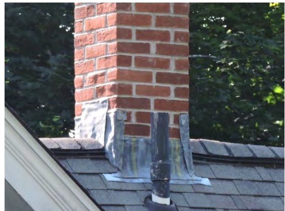
Lead was commonly used for the flashing of brick masonry chimneys and is still present within the historic district.
