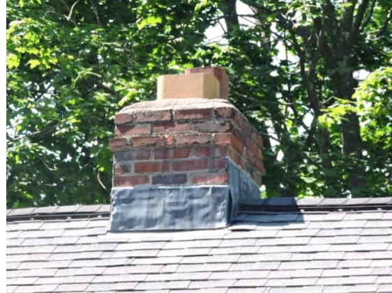
Common utilitarian chimney with original brick, copper flashing, terra cotta flue liners, and cement wash to shed water.
