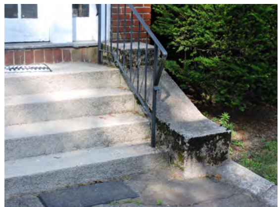
Most metal handrails within the historic district are of modern installation. The posts of metal handrails are susceptible to deterioration where they anchor into concrete or masonry.
