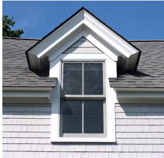
Half dormer flush with the wall and penetrating through the roof in a one-and one-half story cottage.
