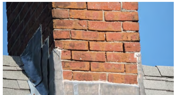
The open joints in this chimney may allow water to penetrate and deteriorate the brickwork.
