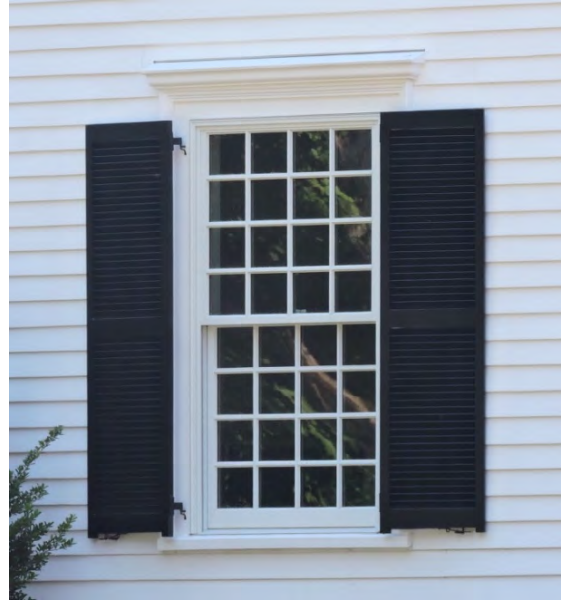
Shutters should match the height and width of the window opening and be operable or at least appear to be operable.
