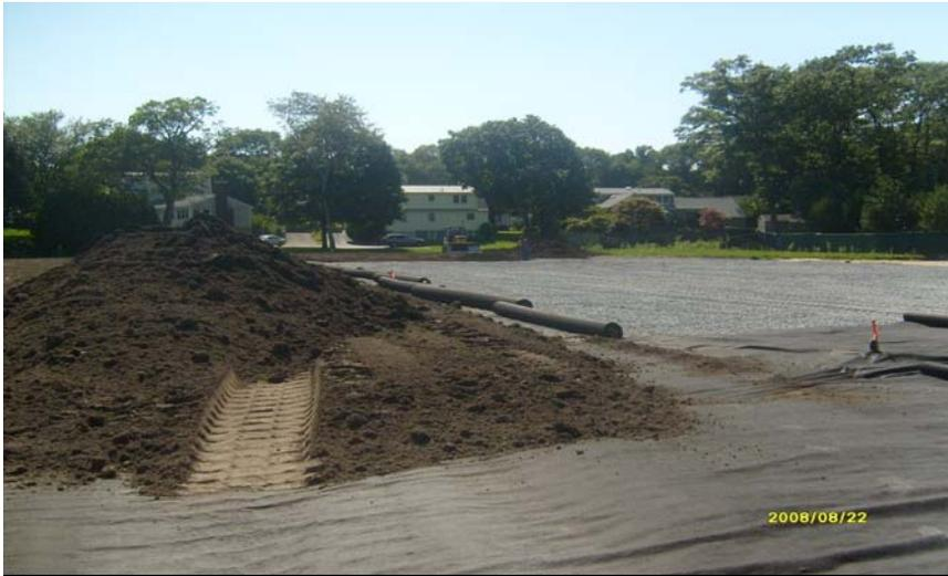
Geotextile Fabric cover with crushed stone
