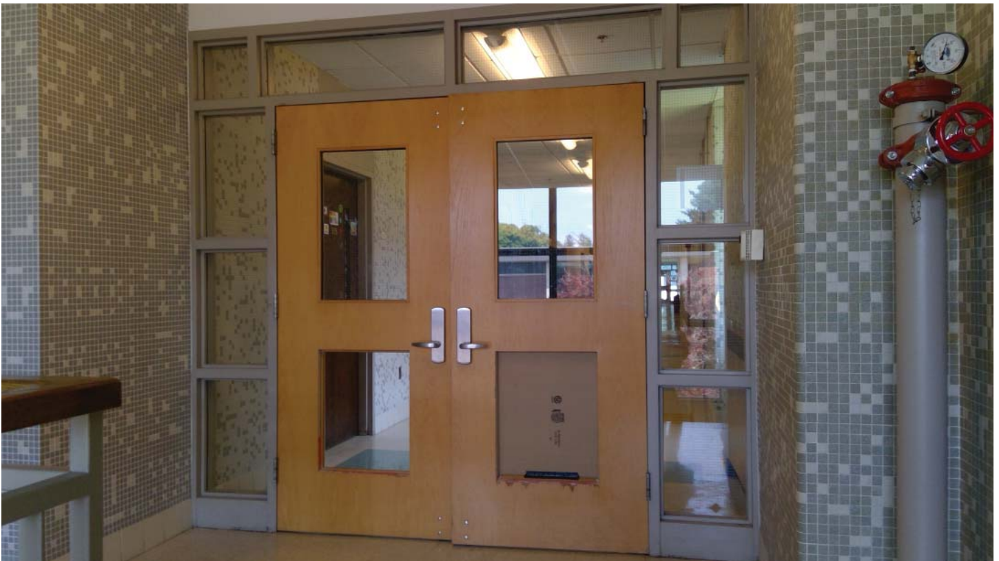
Image 7 - Corridor to Stairs Doors
