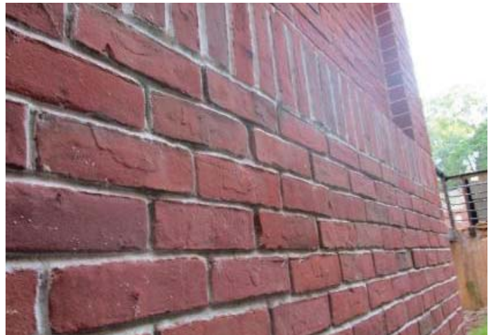
Image 21 – Weathering not affecting 25 yr. service life
