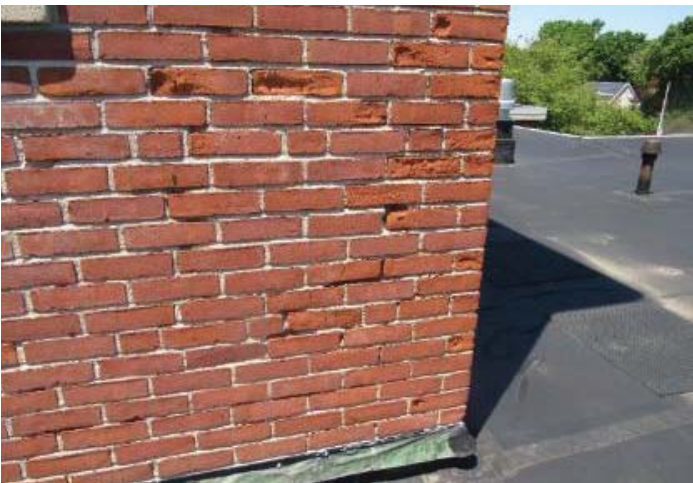
Image 22 – Weathering affecting a 25 yr service life
