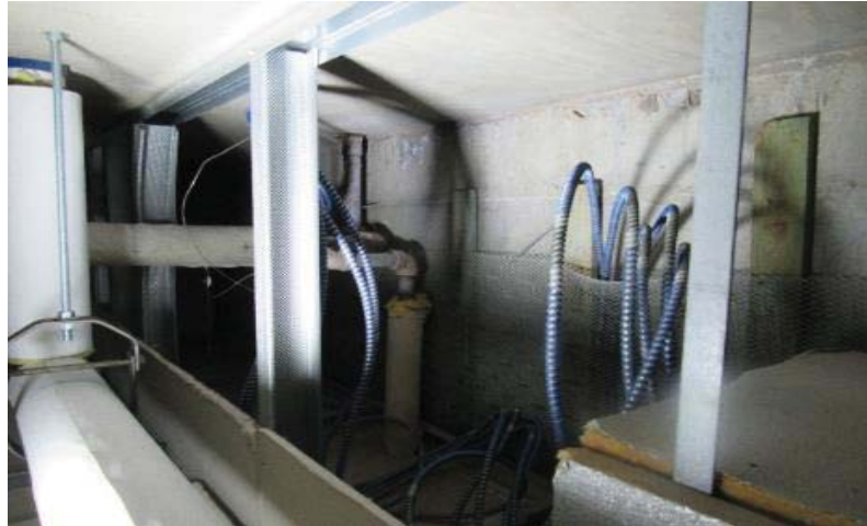
Image 69 – Foundation wall above ceiling tiles
