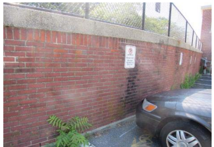
Image 14 – East retaining wall
