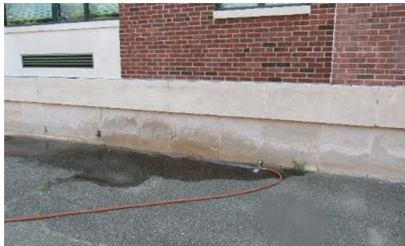
Image 71 – Applied water to base of wall
