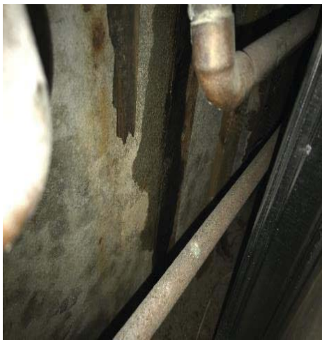
Image 73 – Wetting of the concrete during water test
