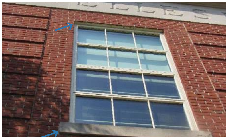
Image 12 – Through-wall flashing at window heads and below limestone sill (arrows)
