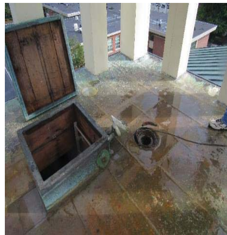
Image 76 – The cupola low-slope roof is accessed through a roof hatch
