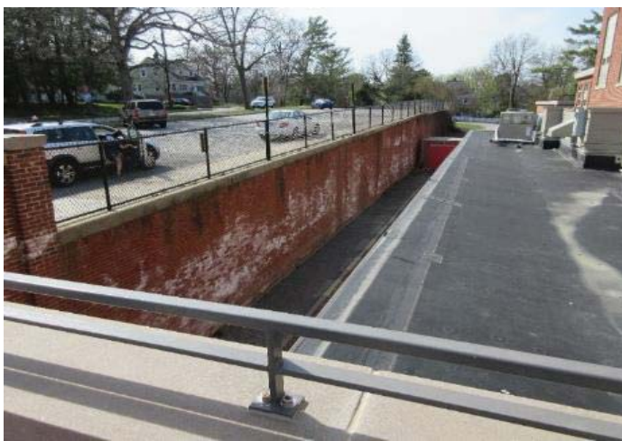
Image 13 – West retaining wall
