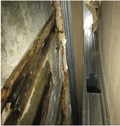
Image 72 – Wetting of the concrete during water test (Image 71, Elevation Sheet 10).
