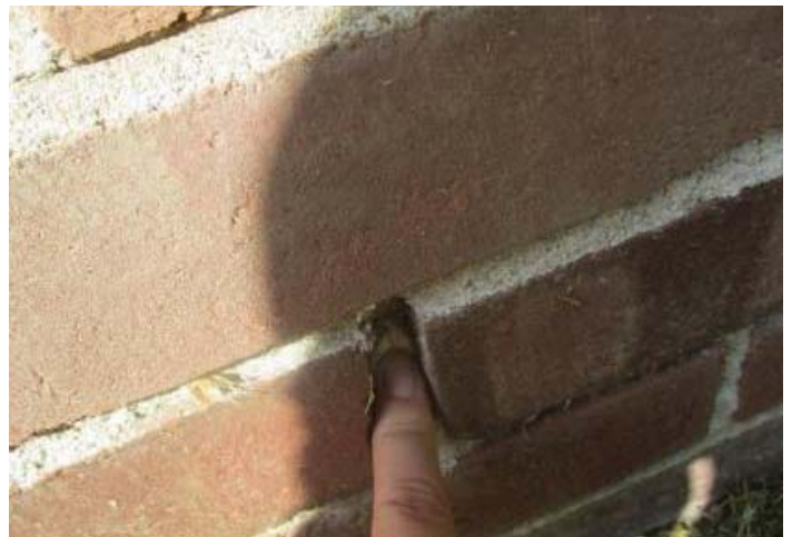
Image 23 – Mortar is white, soft, and powdery to the touch
