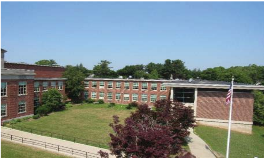
Image 2 - Original 1952 North Courtyard
