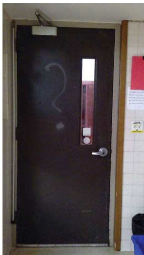
Image 5 - 1966 Classroom to Stair Door
