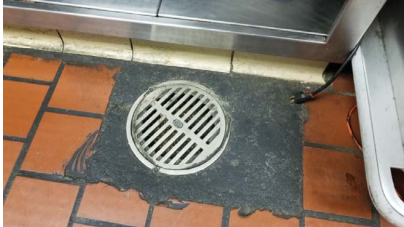
Typical Kitchen Floor Drain
