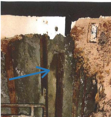
Image 74 – Area during repair (arrow showing location of wetting, Image provided by FMD)
