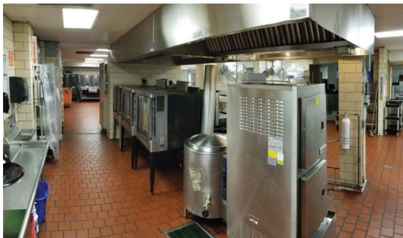
Image 11 - Diffusers in ceiling
