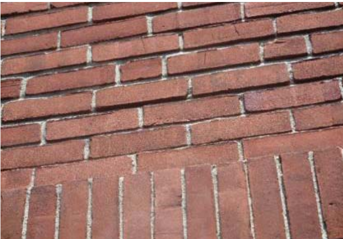
Image 20 – Weathering not affecting 25 yr. service life
