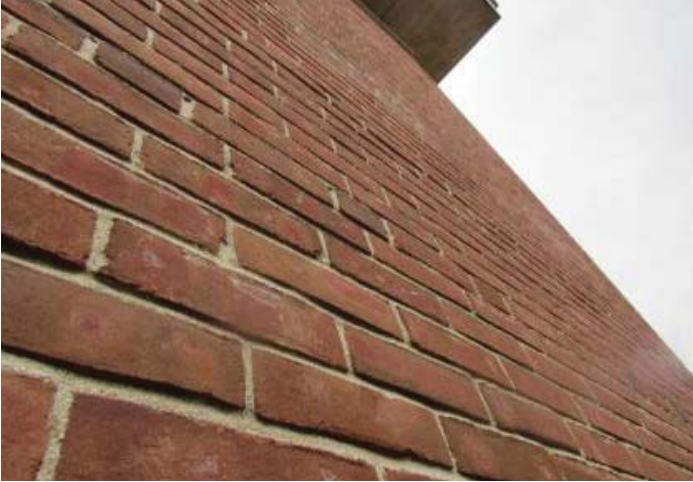
Image 18 – Typical weathering
