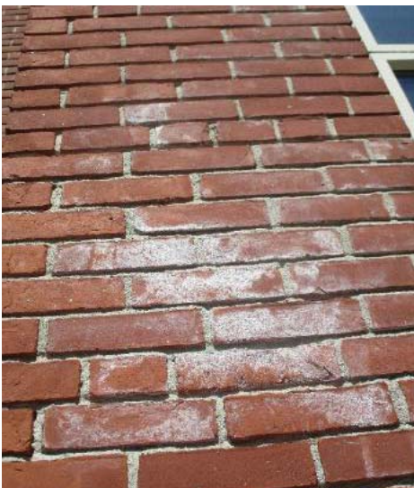
Image 32 – Efflorescence
