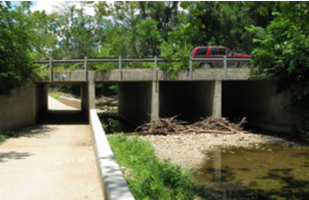
bridge structure in stream channel impedes water flow and is prone to frequent flooding
