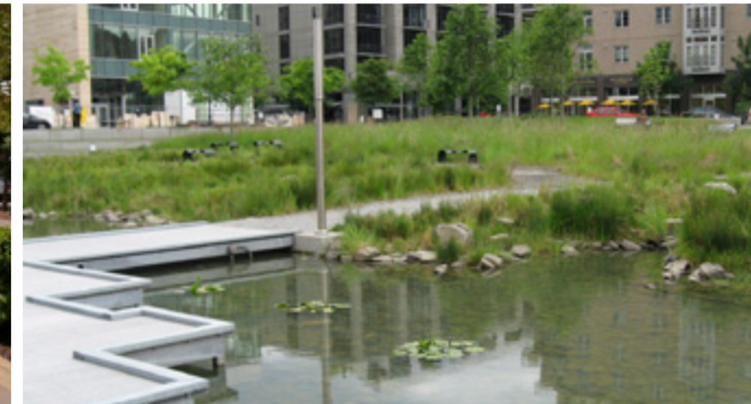
networks: LID networks contain treatment facilities connected to regionally scaled systems of stormwater management.
