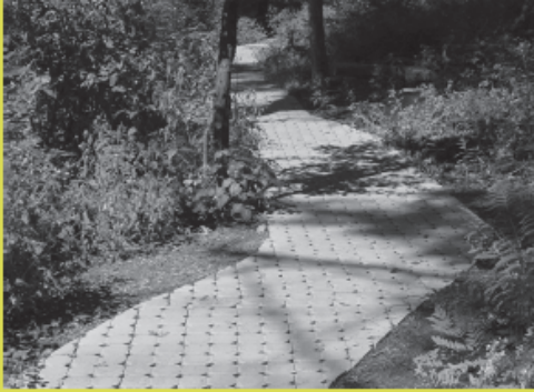
Above: A handicap-accessible park pathway made of permeable paving stones. Photo: GeoSyntec Consultants, Inc.
