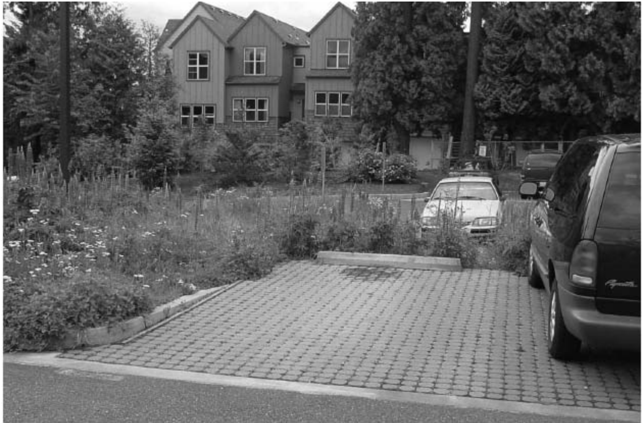
Above: A parking lot with conventional asphalt aisles and paving stone parking stalls. Paving stones are most appropriate for low-speed, low-traffic areas. Photo: Lower Columbia River Estuary Partnership
