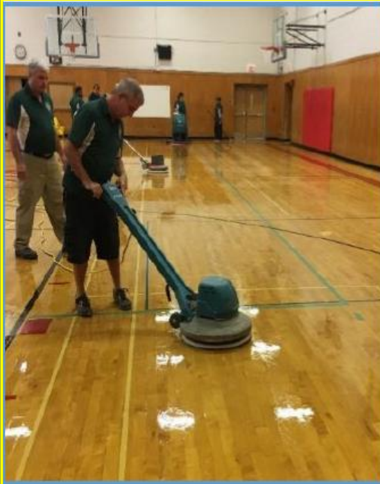
Wet Abrading Process
