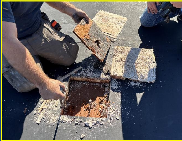
Test Core Sampling
