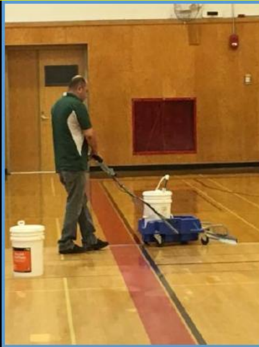
First Coat of Finish Applied
