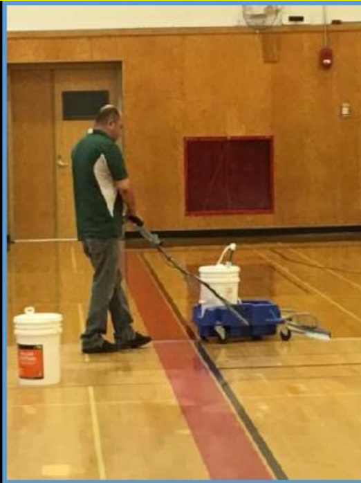
First Coat of Finish Applied
