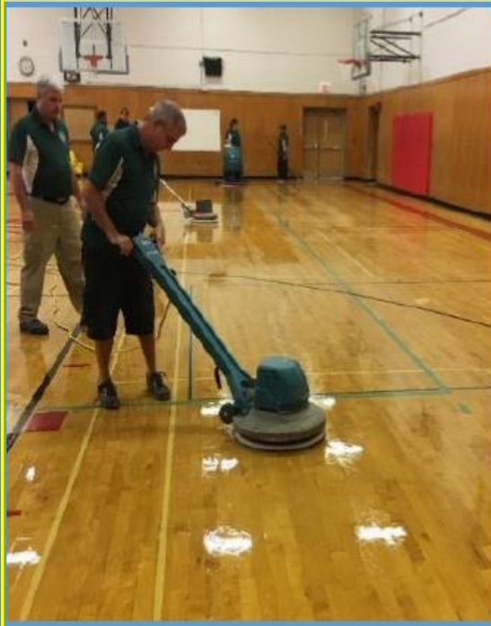
Wet Abrading Process
