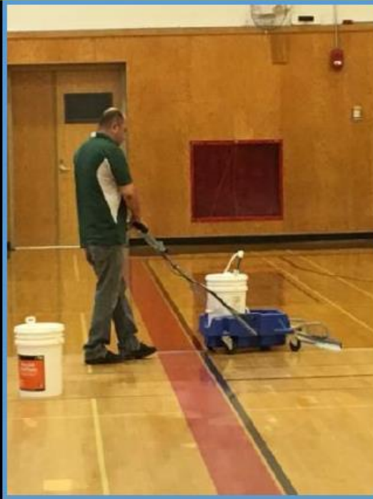
First Coat of Finish Applied
